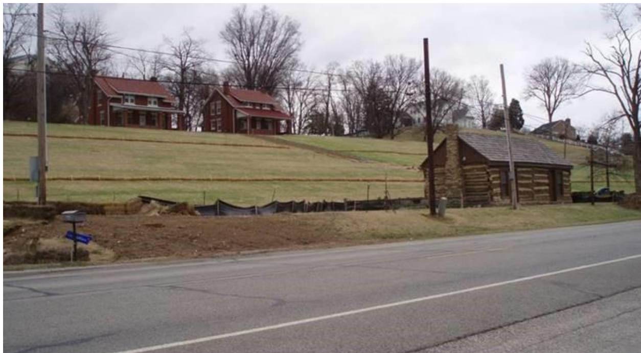
Figure 146. Newburgh Landslide Post Mitigation
